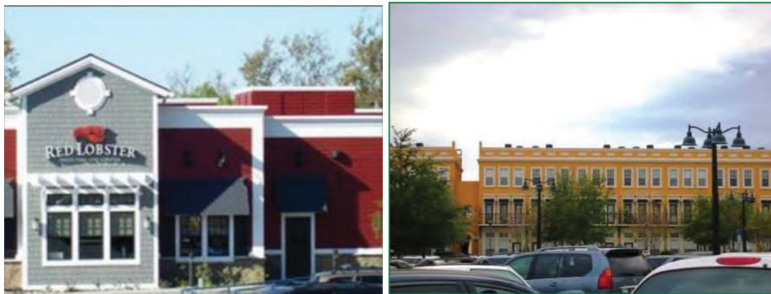
Figure 37. Rooftop Units Screening
