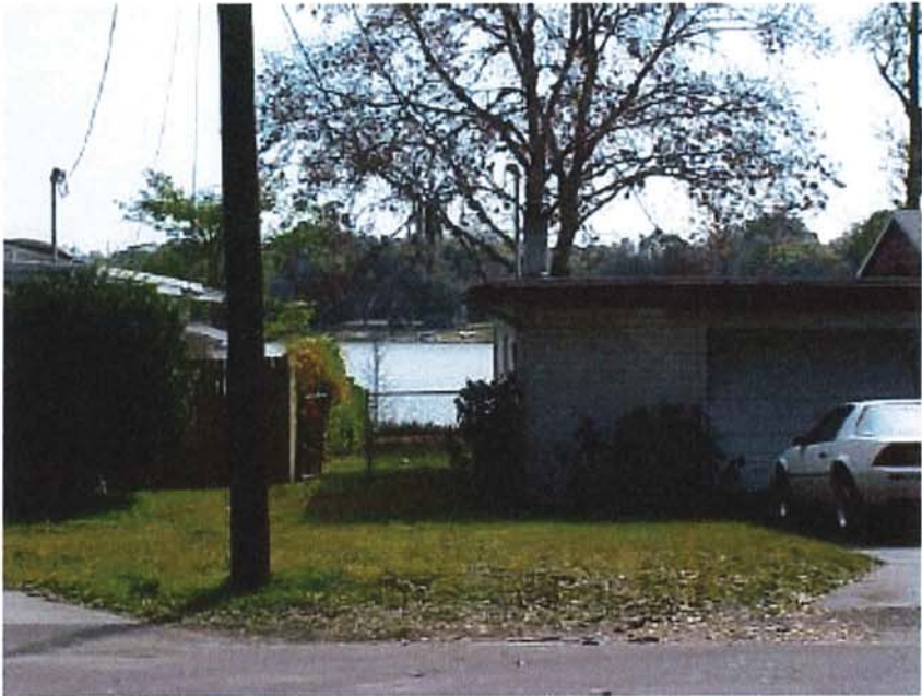
Example of Poor Design with Rear Yards Facing Lake
