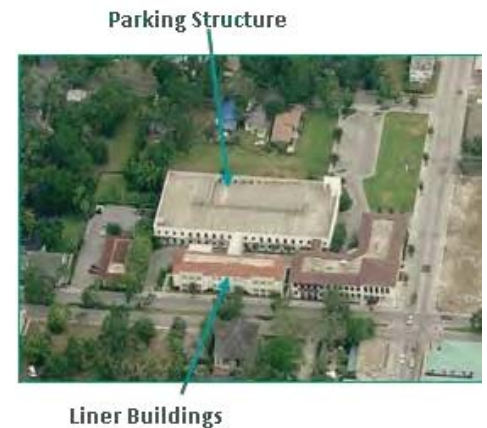
Figure 18. Detached Liner Building
